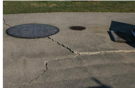
Major crack in pad covering tank and collar
